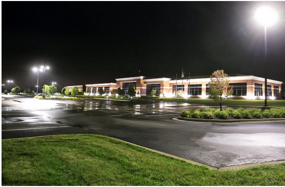
Outdoor car parking lot
